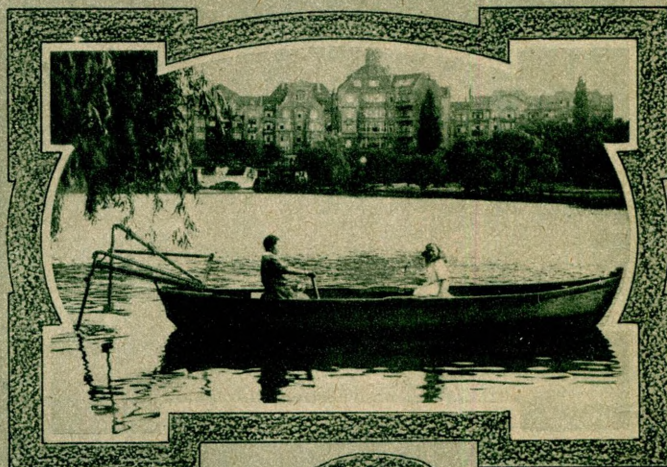
Applying Chlorine Gas at the Kensico Reservoir for Sterilizing the Water Supplied to New York City. The Gas is Received in Liquid Form Comprest in Cylinders. The Croton Supply is Treated Similarly and Smaller Plants in the Catskills and Croton Watersheds Treat the Streams Before Entering the Reservoirs.—(Copyright by Keystone.)
